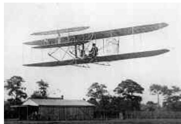
The Wright brothers, Orville and Wilbur, adapted their biplane design from a glider and added a gas powered engine to it. In December 1903 at Kitty Hawk, North Carolina, they succeeded in making the world's first powered, controlled, and sustained airplane flight. Their flight went only 120 ft. at 35 mph but the era of the airplane had begun. They were successful because they were the first to develop a method for control.
