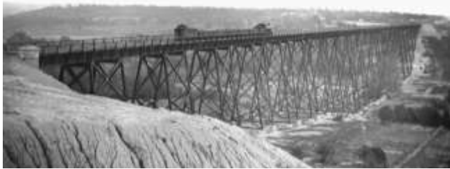
Original Honey Creek Bridge
